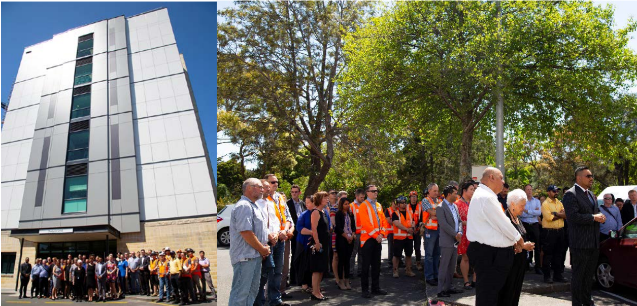
Pictured above: Counties Manukau Health and Hawkins staff marking the end of Re-clad Stage 1
