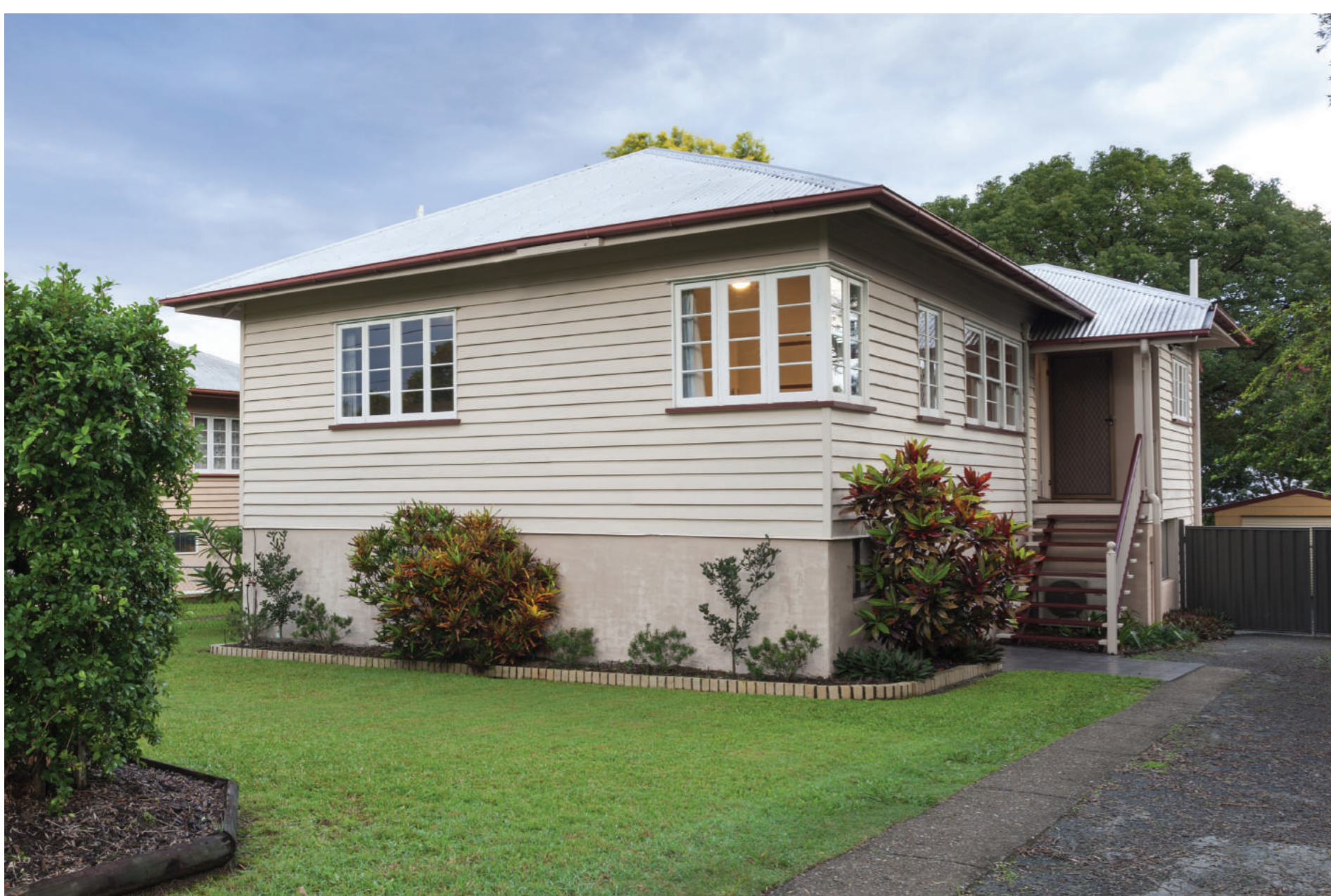
Many homes in New Zealand built between 1940s and 1980s were built using products containing asbestos
