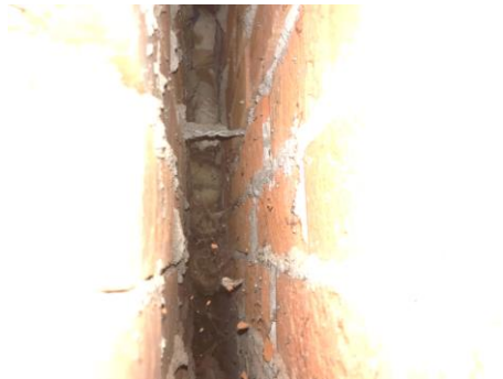
Packing in the distance used as form for internal column
