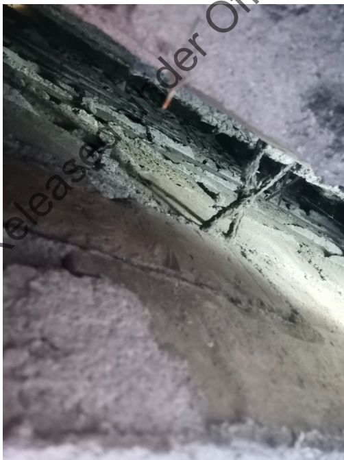
Figure 2: Evidence of cavity ties in external walls
