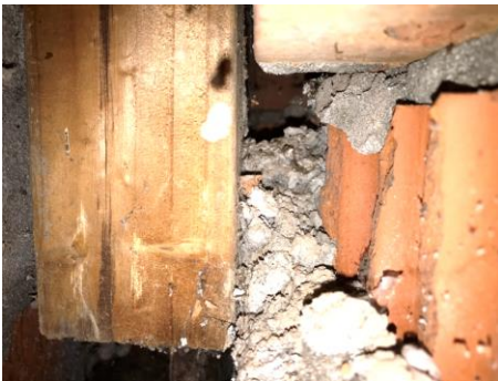
Timber form, however column not apparent behind
