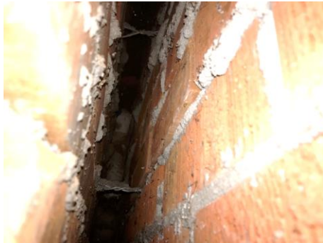
Evidence of packing formwork in distance
