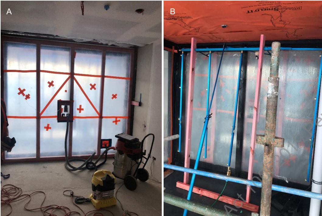
Figure 3: Example pressure box test set up, A interior, B exterior
