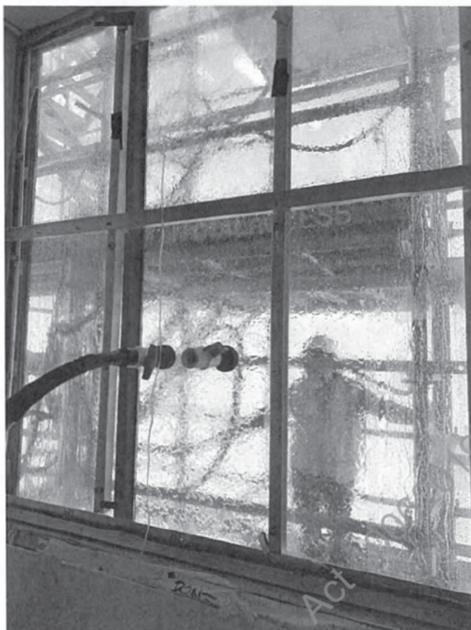
Figure 4: Unit 2 testing from inside with vacuum and pressure measurement tubing attached to acrylic surround
